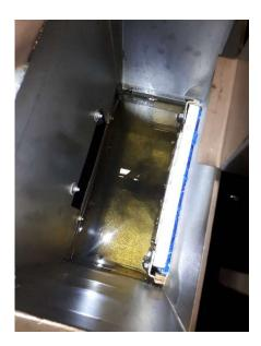
Figure 12. PAC escaping through the pile cloth filter after backwash.
